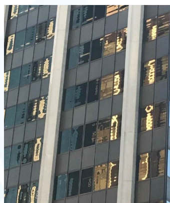
Roller wave is most visible on reflective glass
